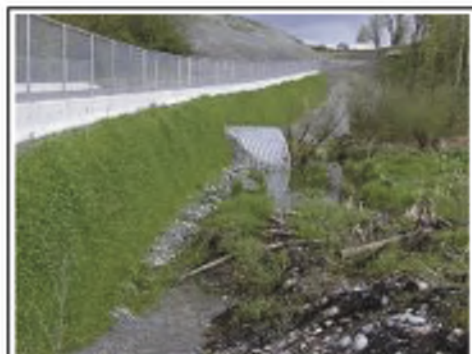
Vegetated Culvert Headwalls
